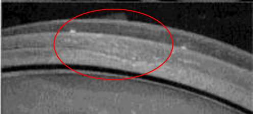
Fig. 8: Irregular contact surface on the edge of tyred wheel rim
